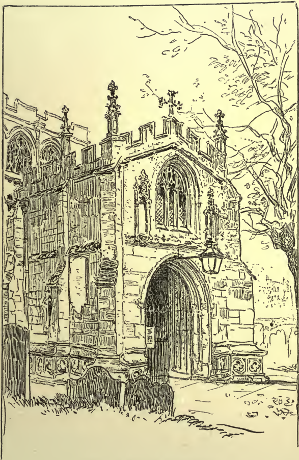
PORCH OF STRATFORD CHURCH.
